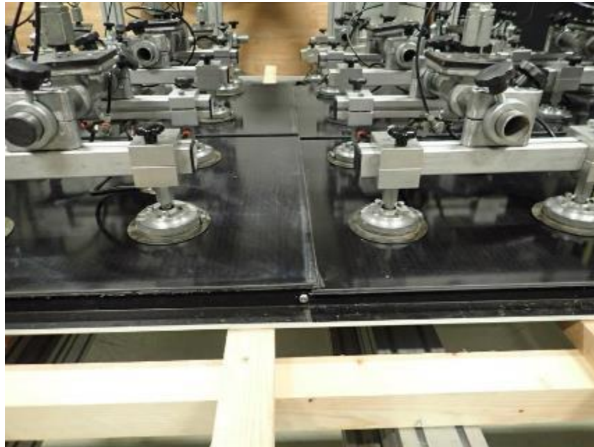
Fig. 5: details of installed system prior to start testing
