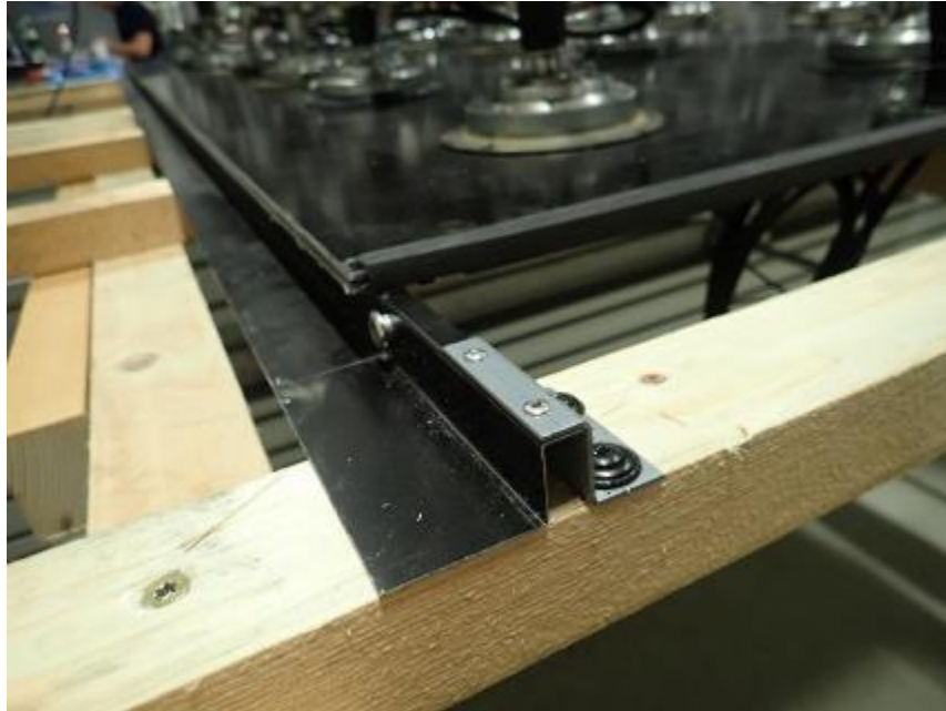
Fig. 3: details of installed system prior to start testing
